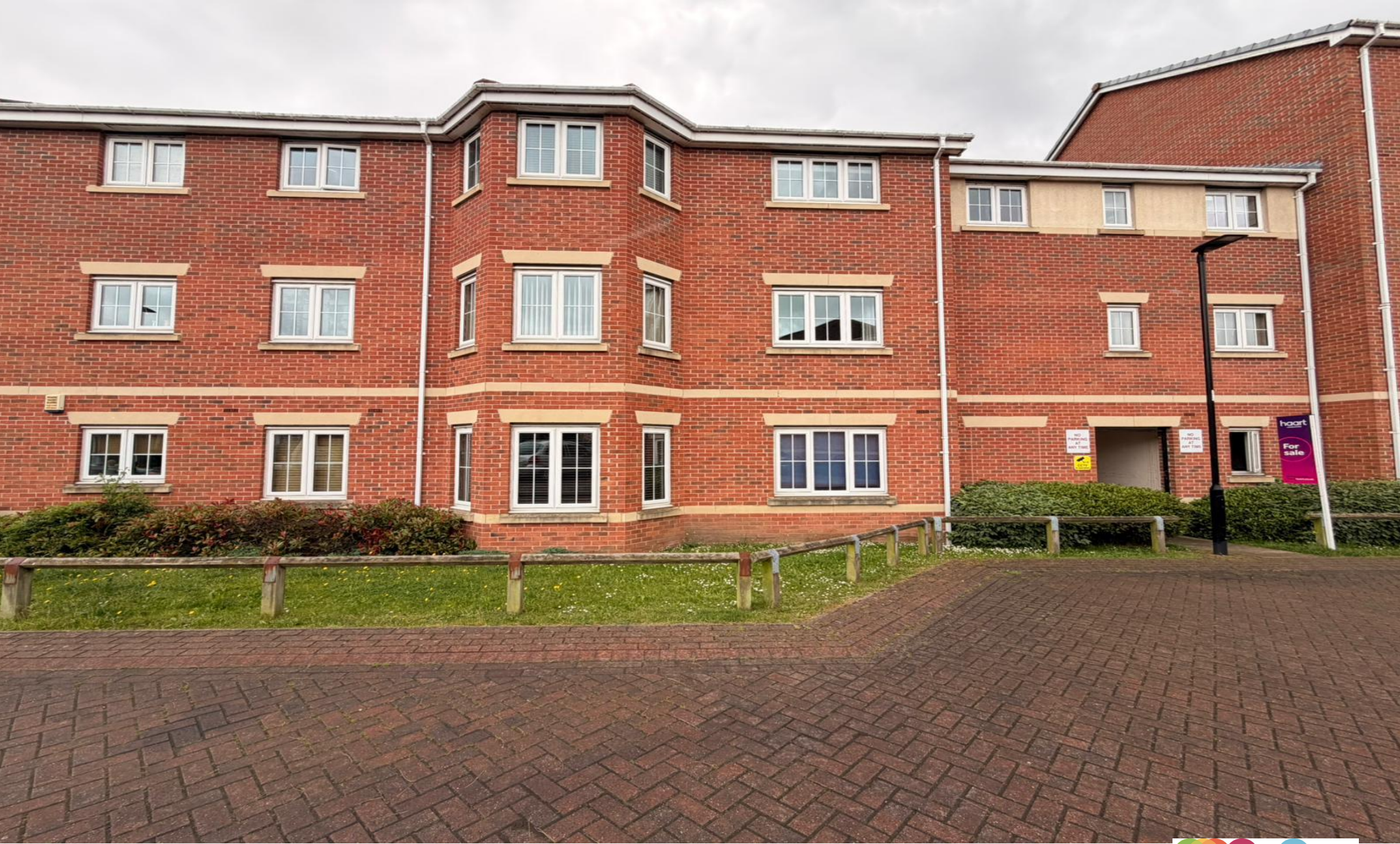
Jenkinson Grove, Armthorpe Doncaster
