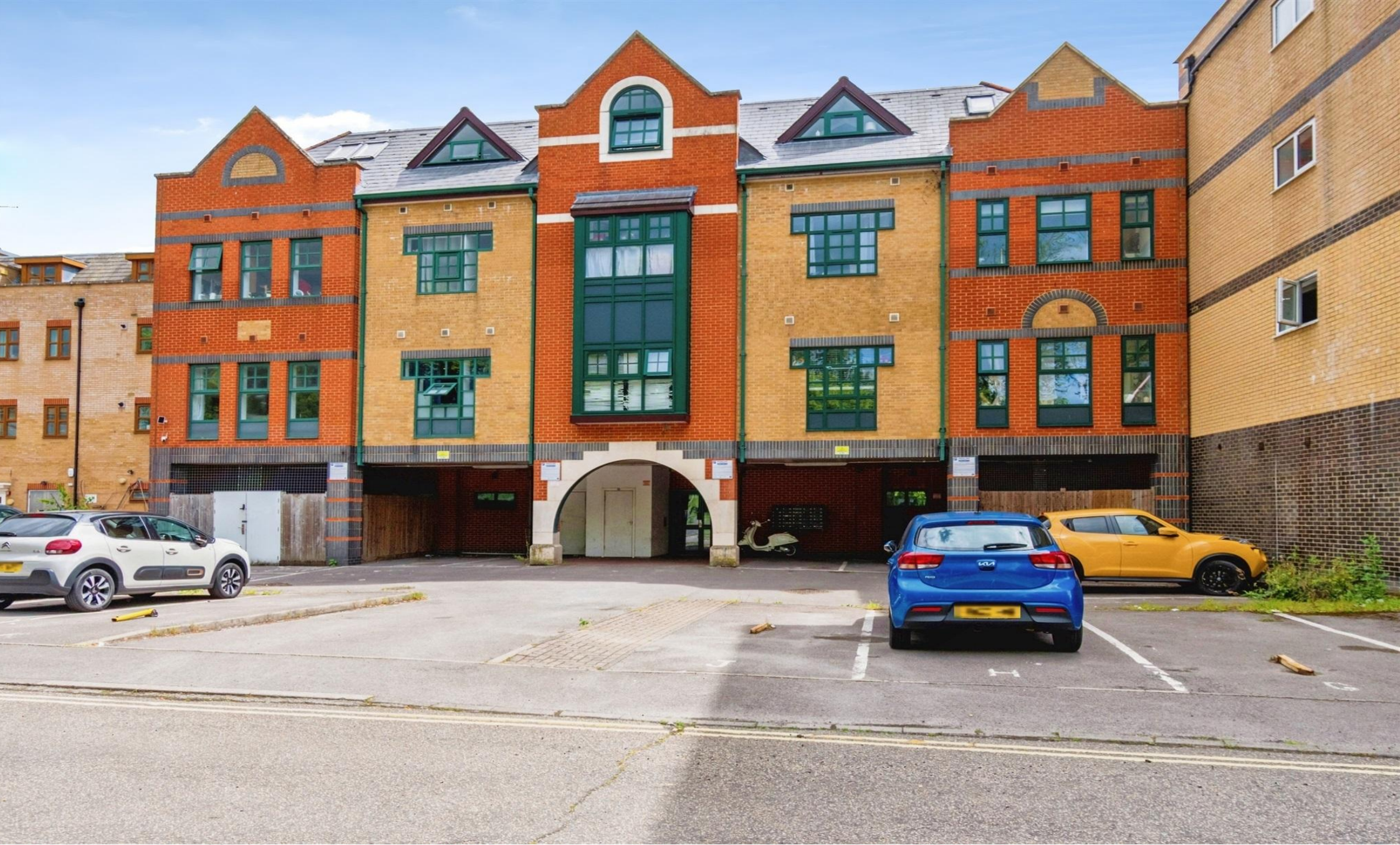
Hampton House, St. Marys Place, Southampton SO14 1AZ
