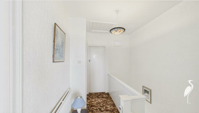
Radiator and access point to loft.
