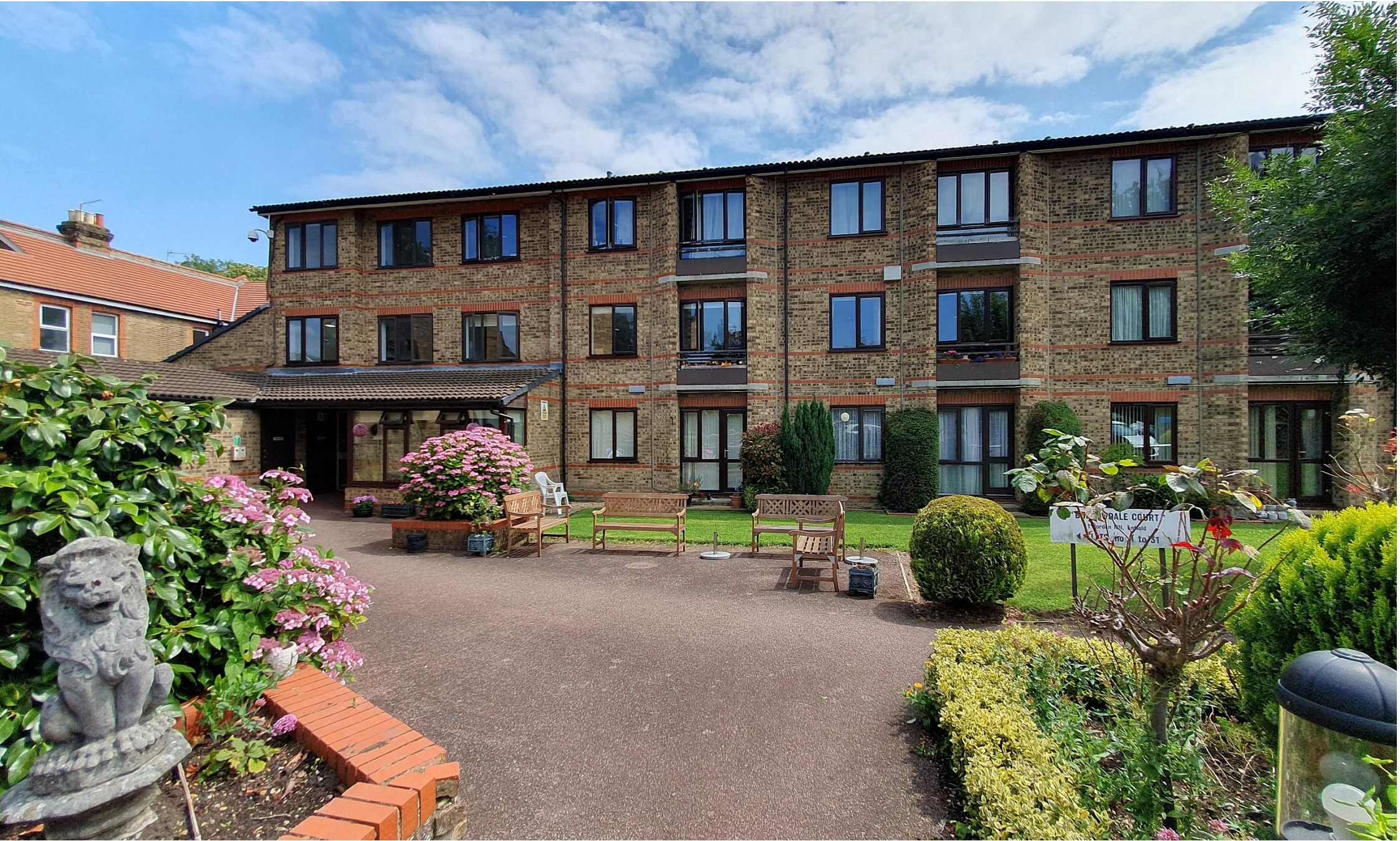
Borrowdale Court Gordon Hill, Enfield EN2 0QJ
