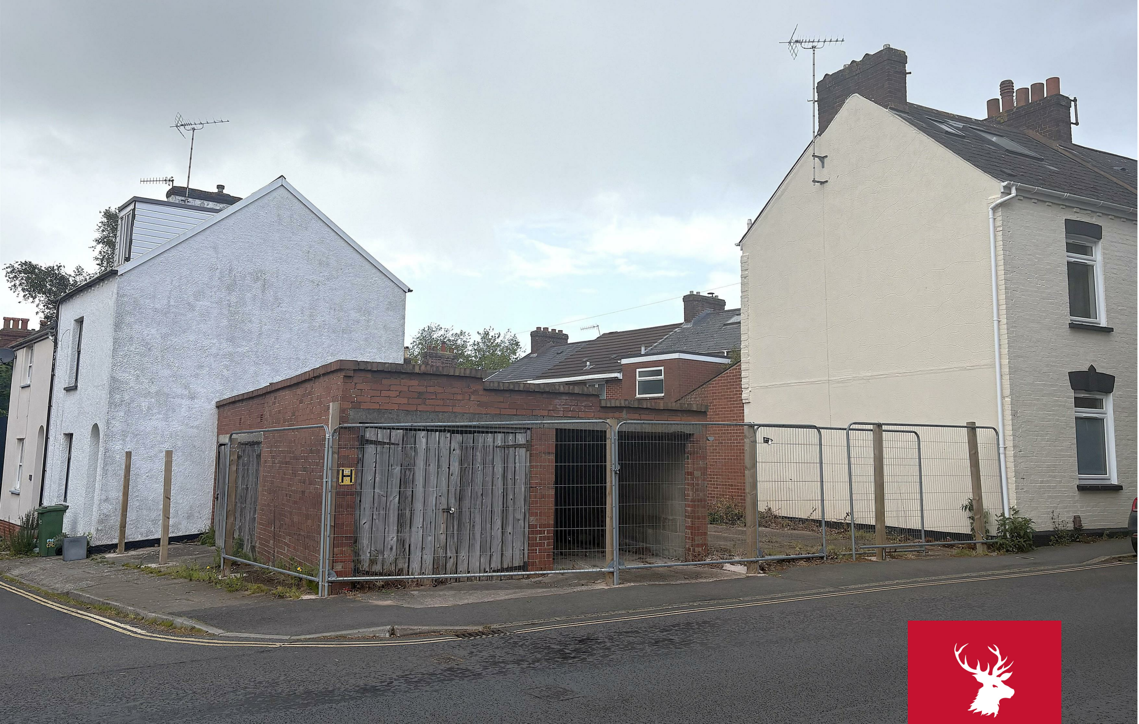
Development Site at Gladstone Road
