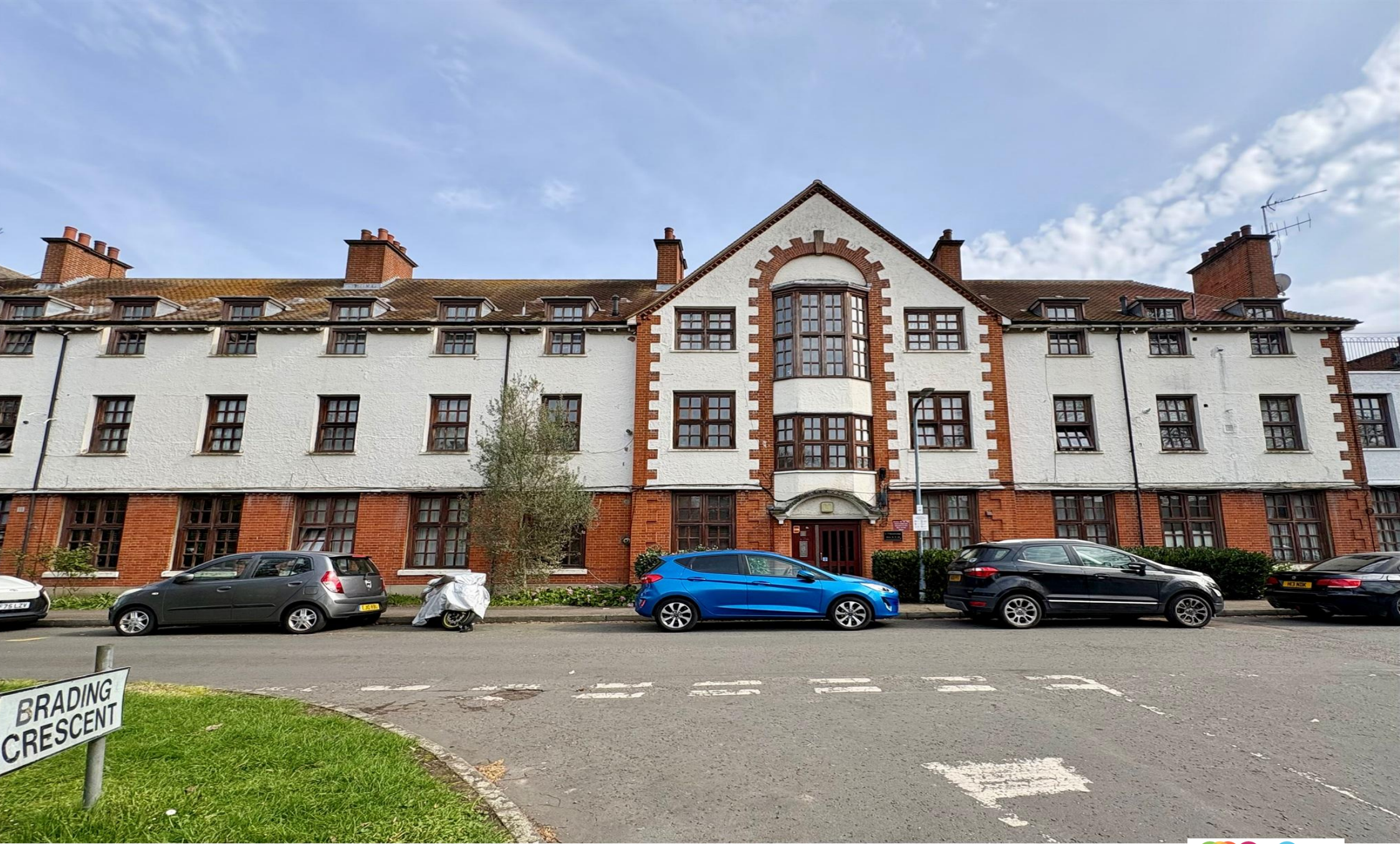
Hood Lodge, Brading Crescent, London, E11 3RW
