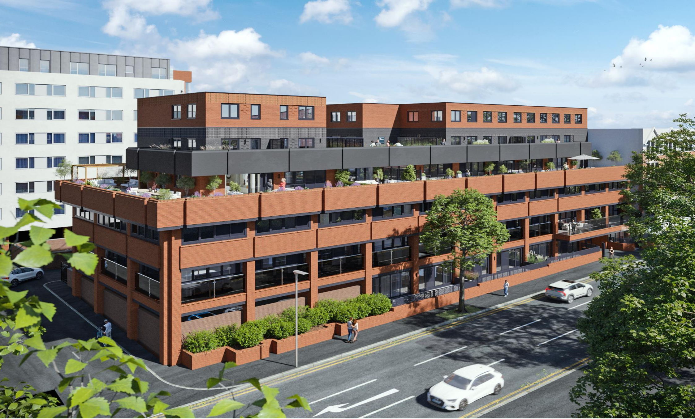
Preece House Davigdor Road, Hove BN3 1RE
