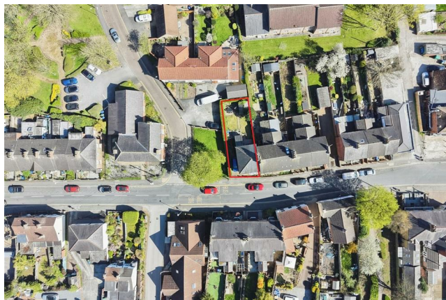
Aerial view of the property
