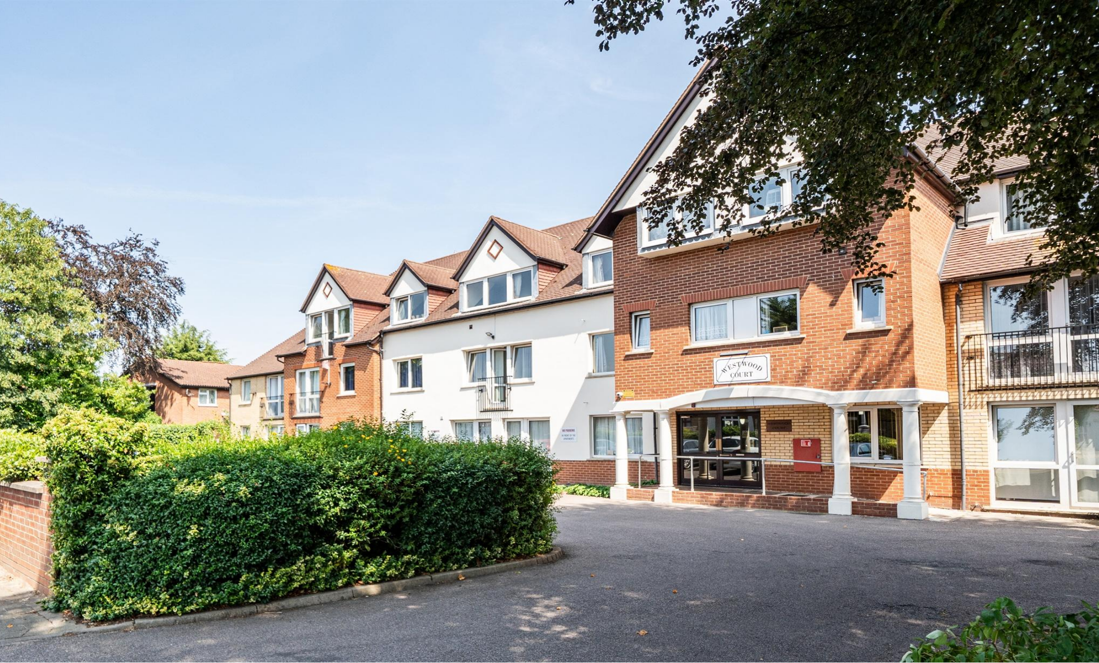
Westwood Court, Village Road, Enfield, EN1 2HQ
