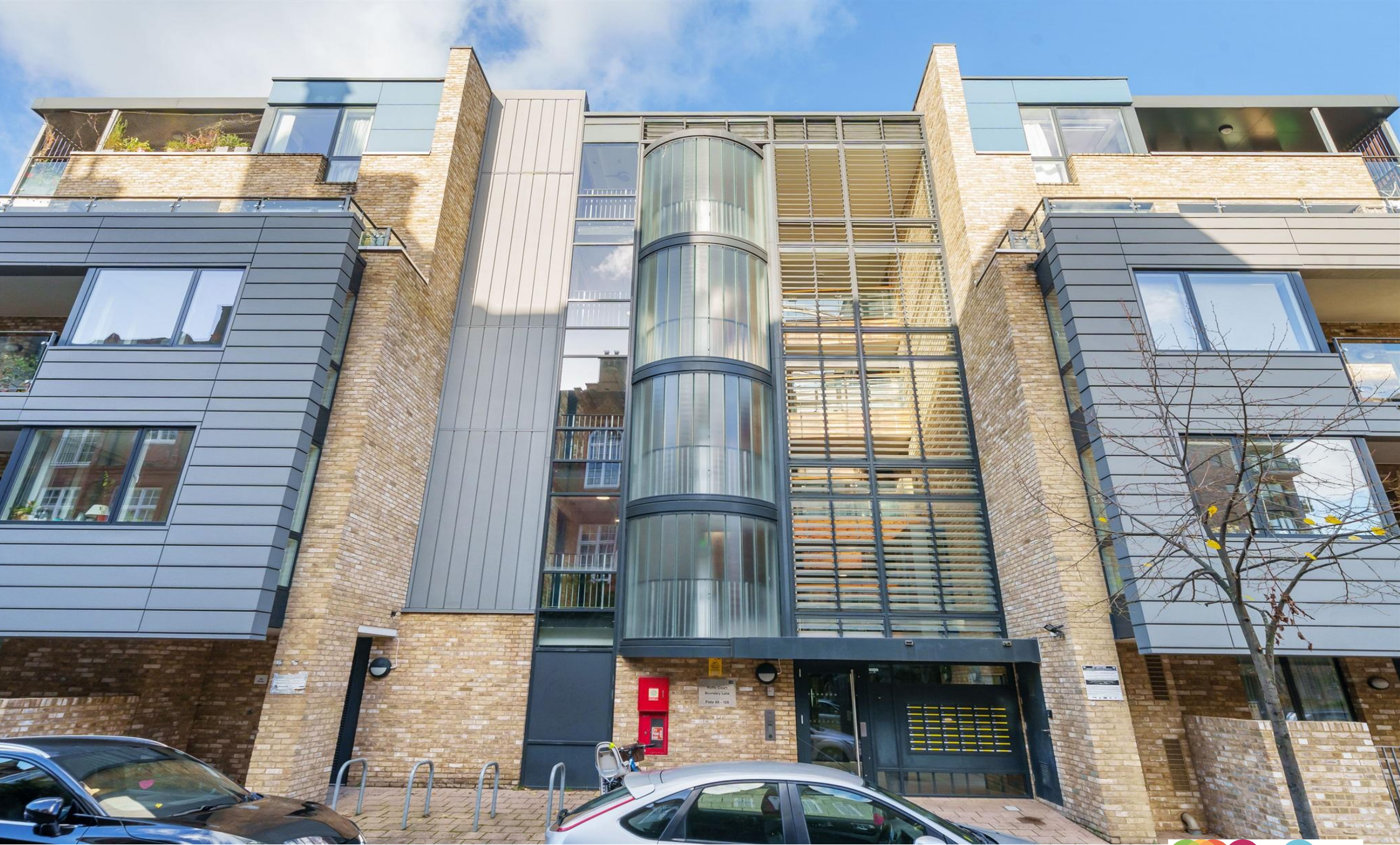
Roffo Court Boundary Lane, London SE17
