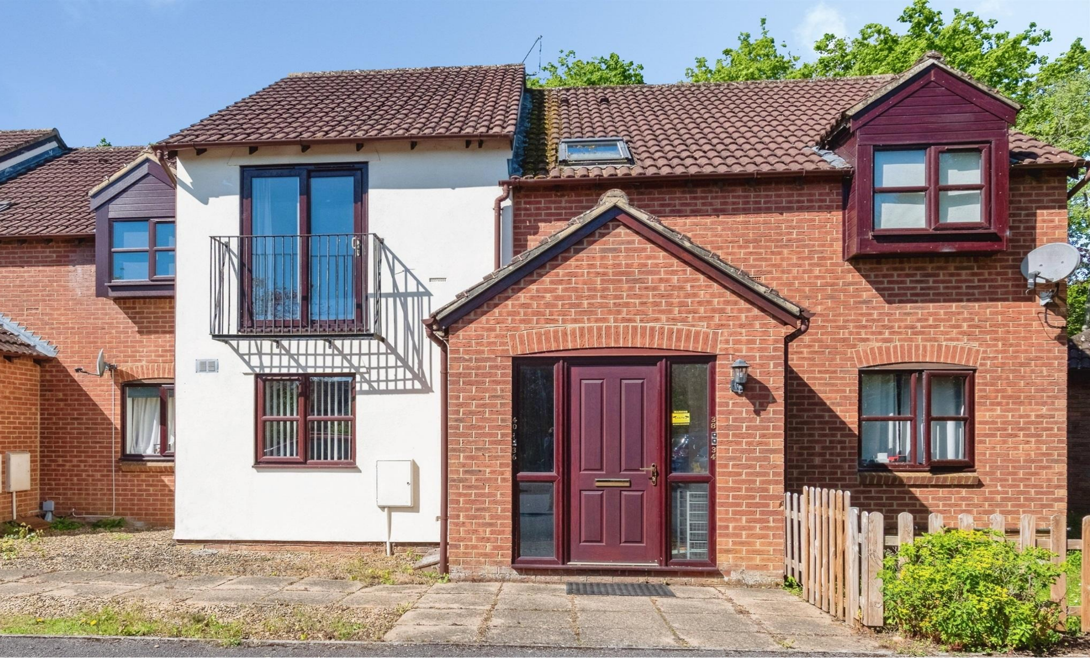
Warwick Close, Chippenham SN14 0YD
