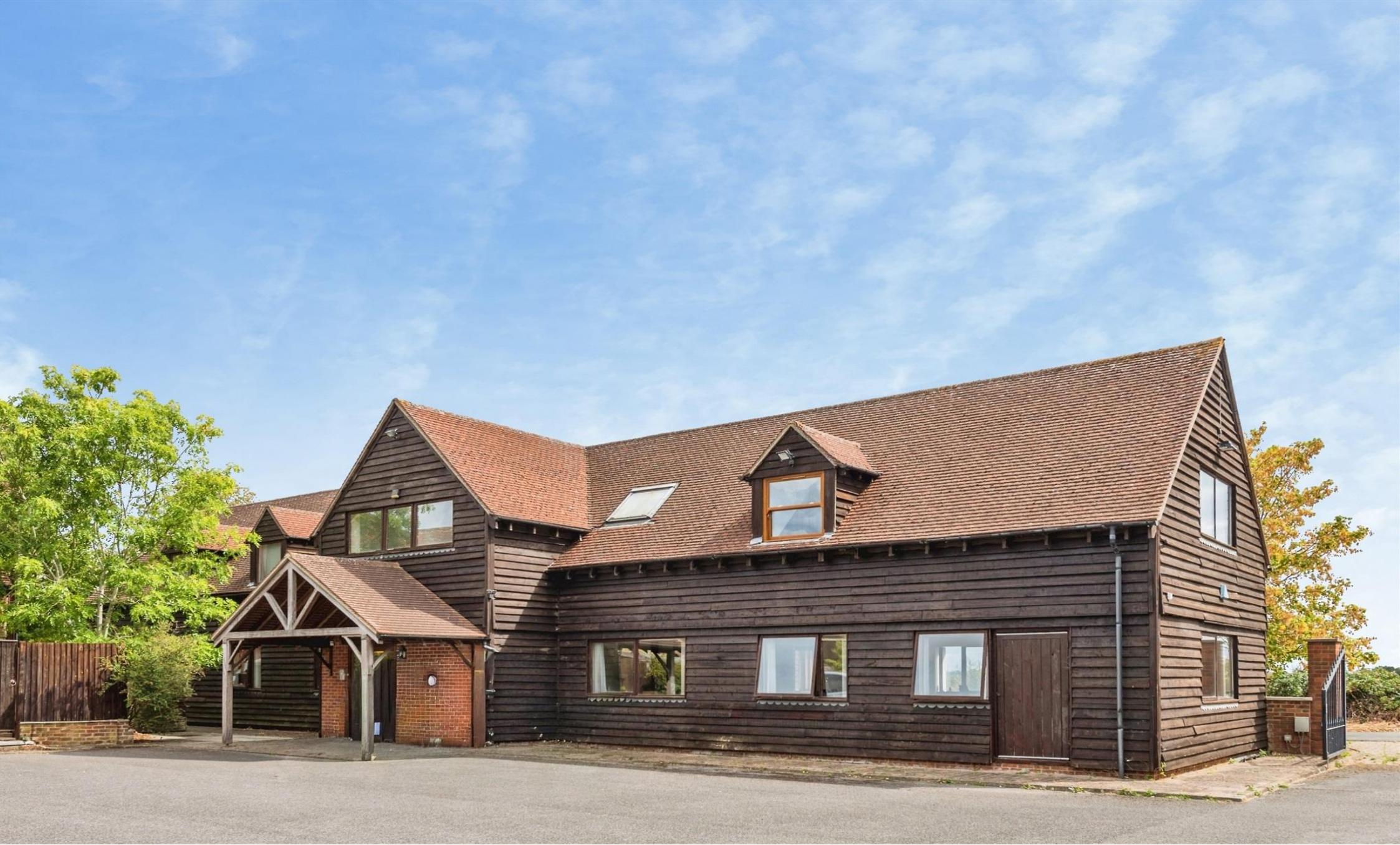
The Office Barn Sugworth Lane, Radley, Abingdon, OX14 2HX
