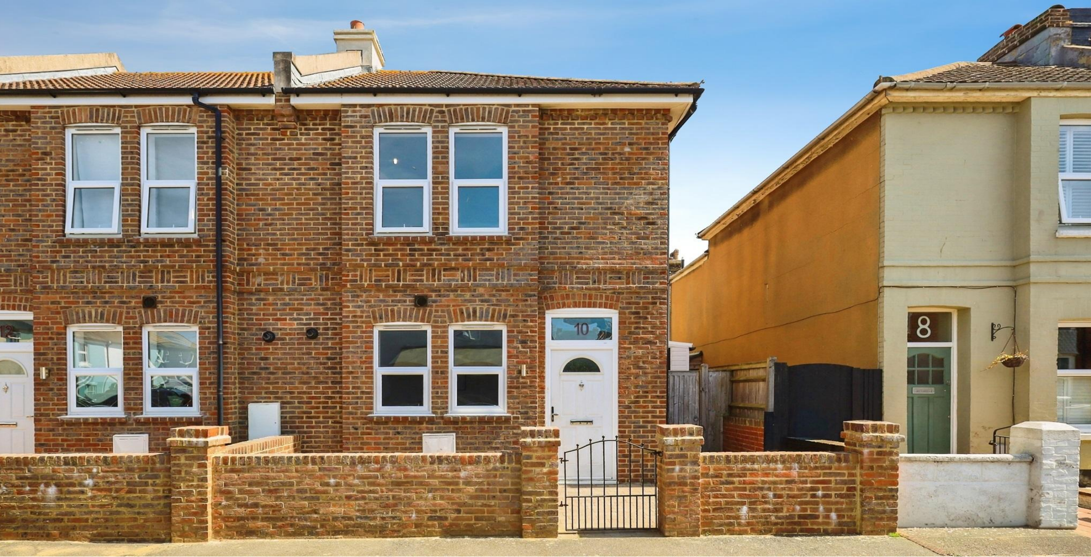
Fairlight Road, Eastbourne BN22 7NY
