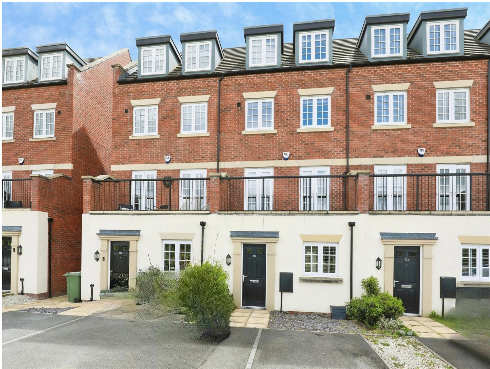
Curzon Avenue,NORTHWICH CW8 4YU
