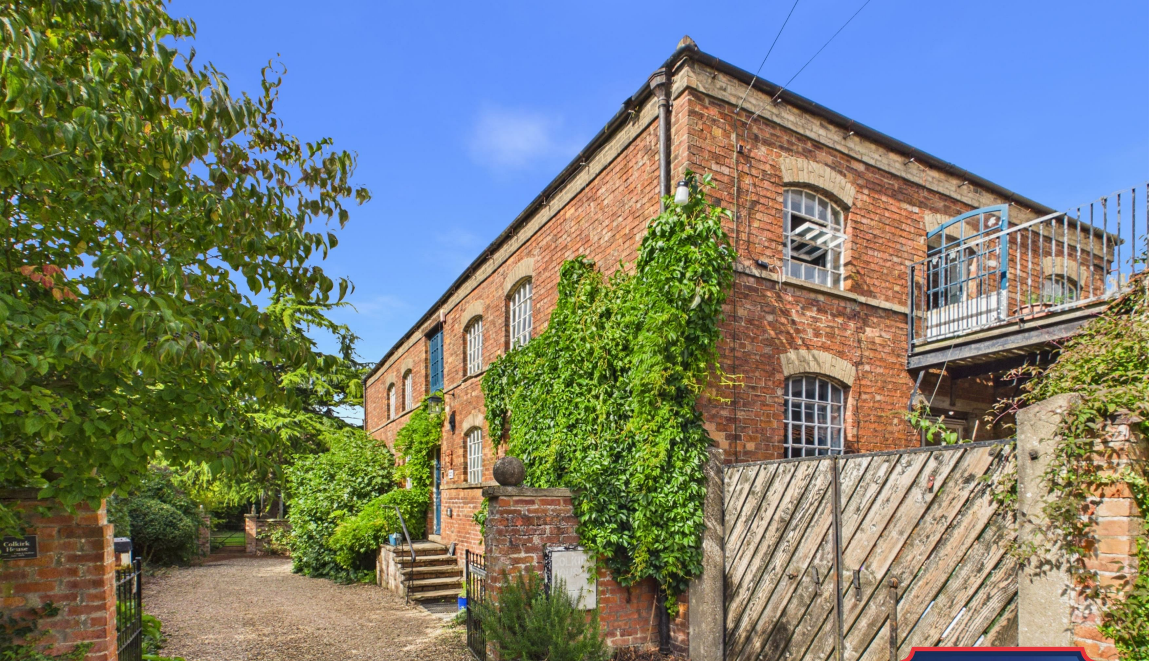
Colkirk House, Manor House Street Horncastle, LN9 5HF
