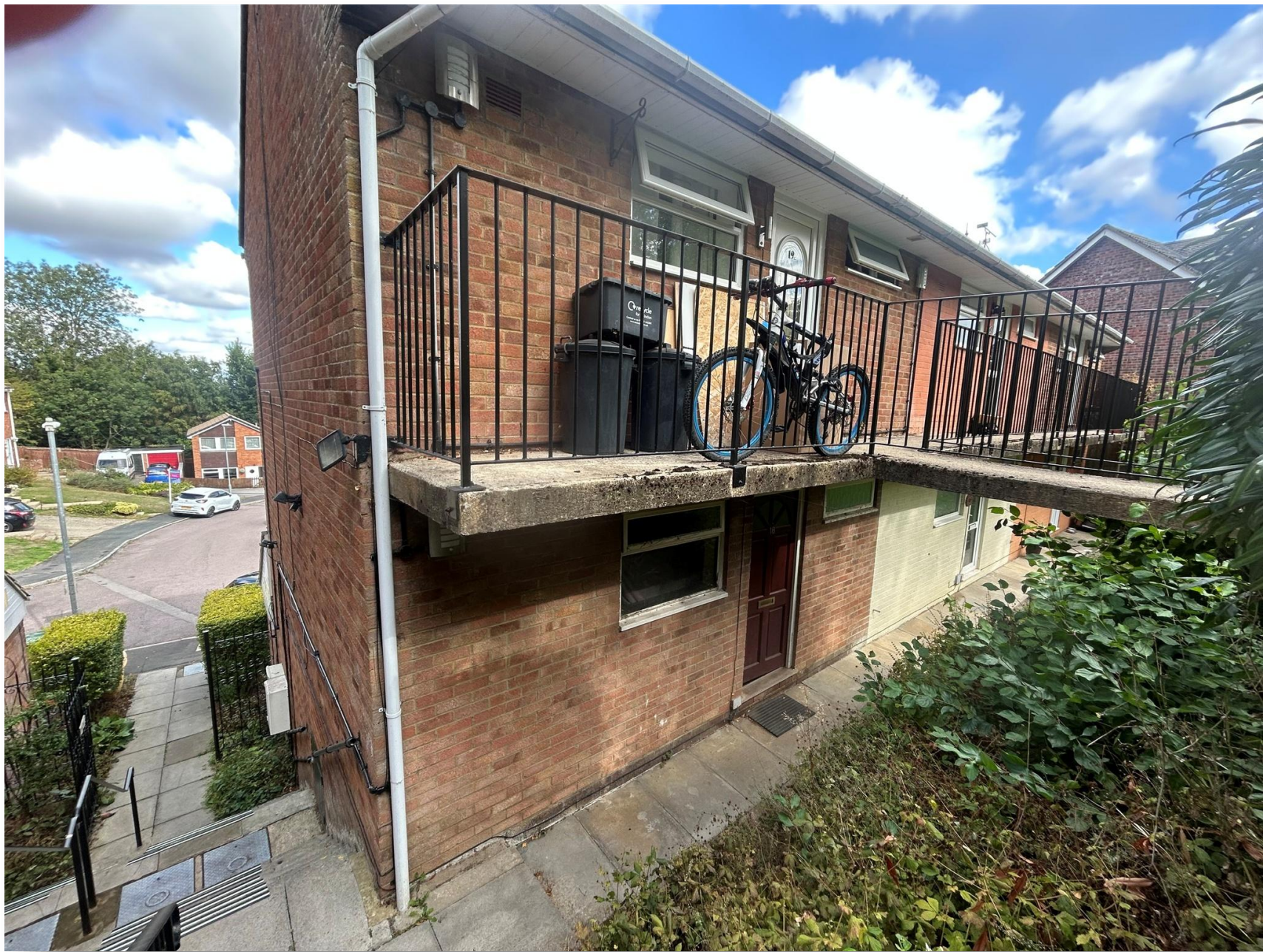
Valleyside, Swindon SN1 4NB
