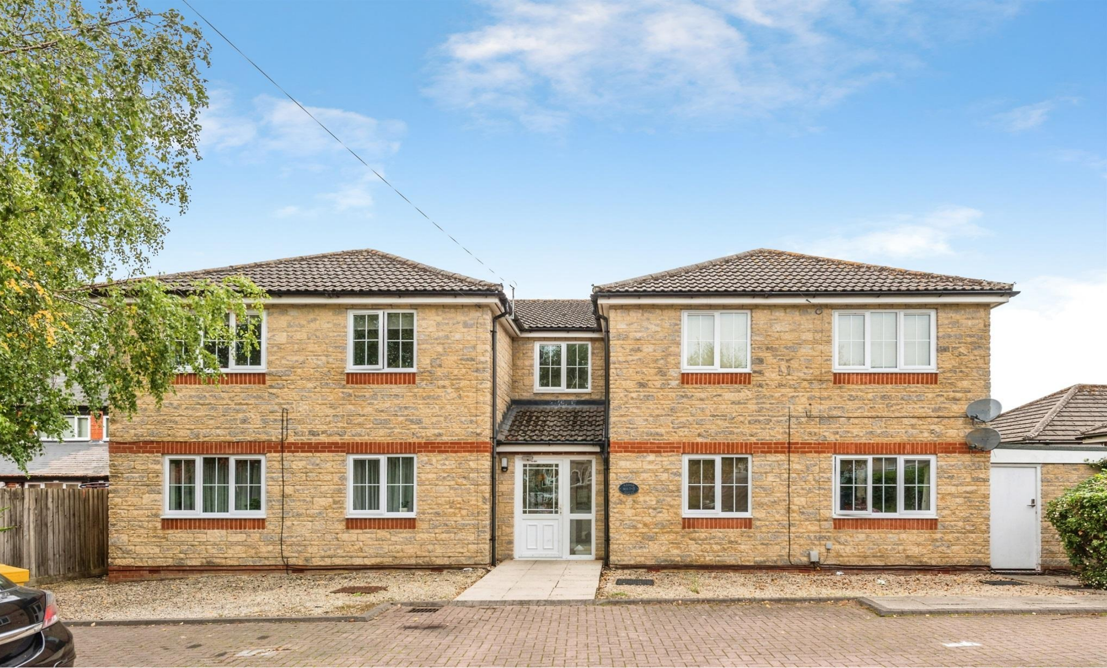
Keogh House, Cheney Manor Road, Swindon, SN2 2PE
