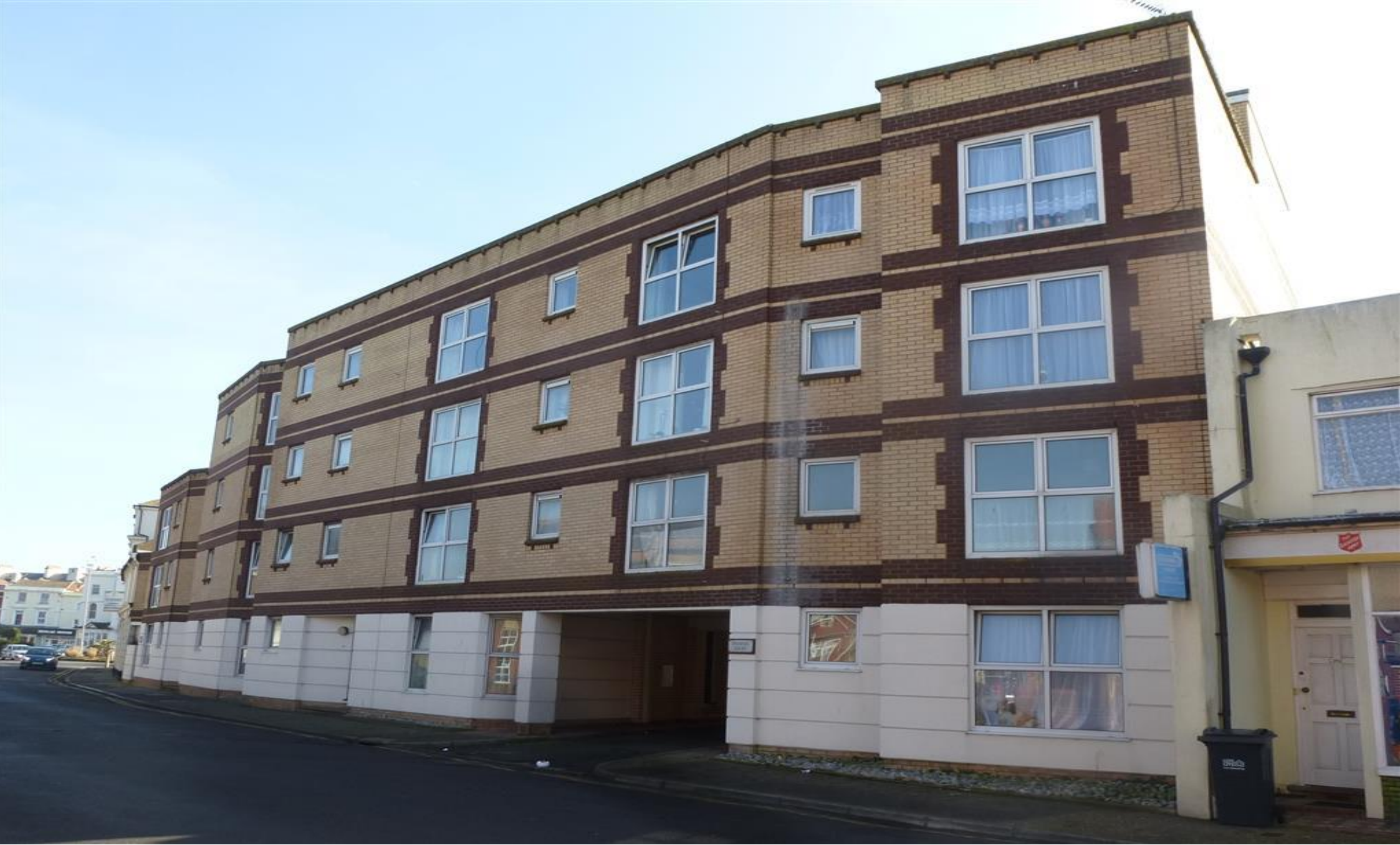
Phoenix Court Langney Road, Eastbourne BN22 8AJ
