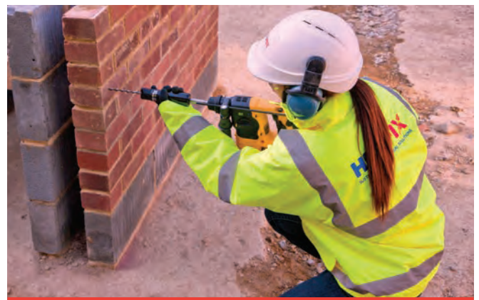
DryFix tie being power-driven into pilot hole
