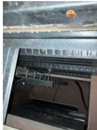
Compartment wall not completed
