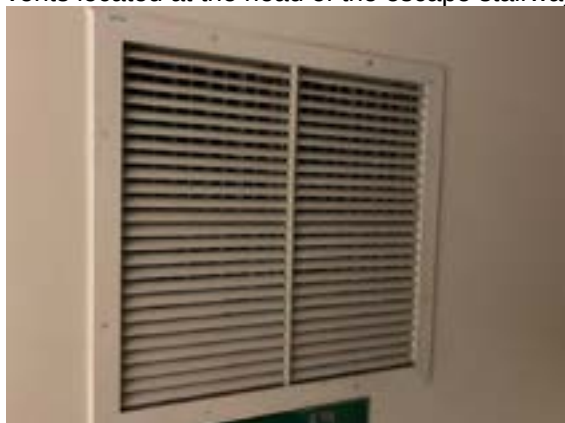
Vent in Stairwell/Escape Route
