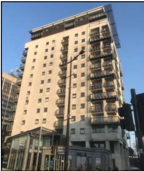
Figure 5.3 : (Left) South-West and Part North-West facing elevations to The Aspect consisting of Render and Timber Cladding Panels and balconies. (Right) North-East and Part North-West facing elevations to The Aspect consisting of Render and Timber Cladding Panels and balconies.
