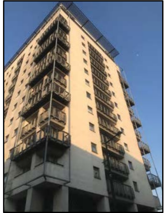
Figure 5.2: (Left) Part South-East facing elevations to The Aspect consisting of Render and Timber Cladding Panels and balconies. (Right) South-West and Part North-West facing elevations to The Aspect consisting of Render and Timber Cladding Panels and balconies.
