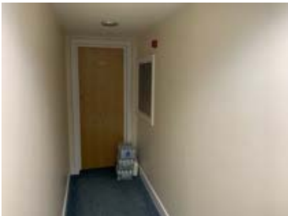
Item(s) in Escape Route
