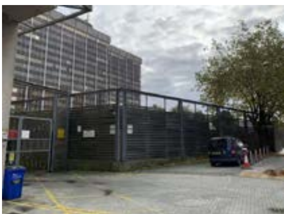
Multi-Storey Car Park
