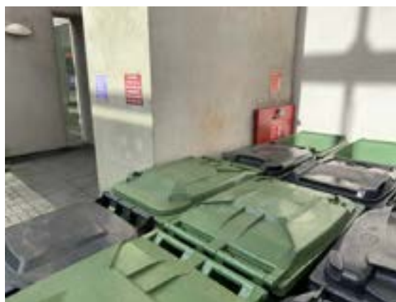
Dry Riser Inlet
