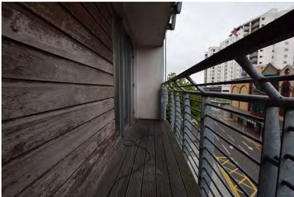
Figure 12 – Example of balcony
