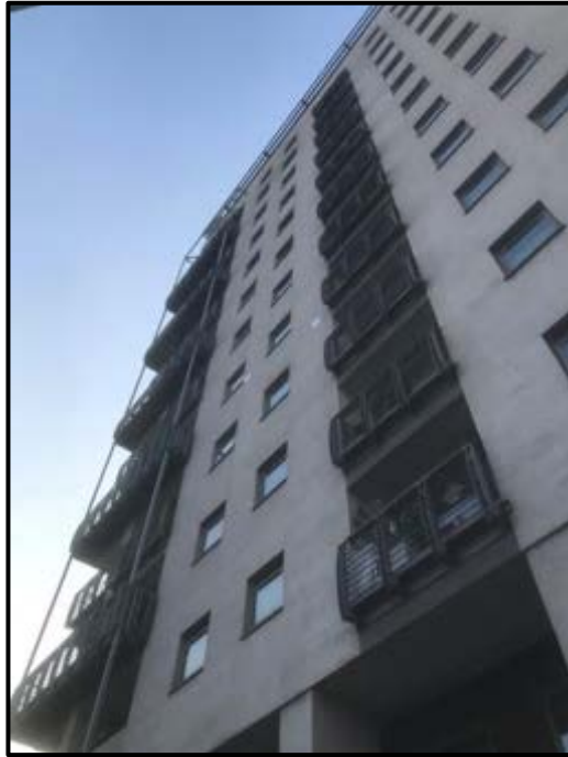
Figure 5.2: (Left) Part South-East facing elevations to The Aspect consisting of Render and Timber Cladding Panels and balconies. (Right) South-West and Part North-West facing elevations to The Aspect consisting of Render and Timber Cladding Panels and balconies.
